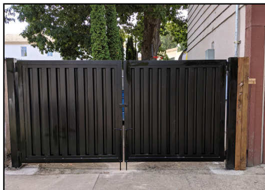
New gate for dumpster area and back yard.
