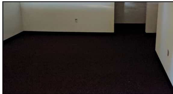
New carpeting in Room 10.
